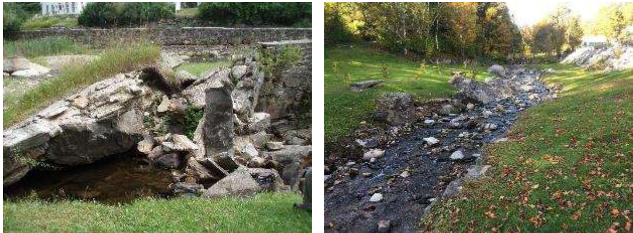
Figure 23. Weston Dam breached in Tropical Storm Irene (before and after removal)
