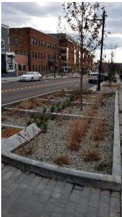
Figure 13. Example of a Green Stormwater Infrastructure Practice, a gravel wetland on St. Paul Street, Burlington completed in 2019.
