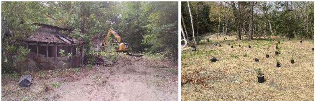
Figure 24. Damaged abandoned buildings and subsequent floodplain restoration
