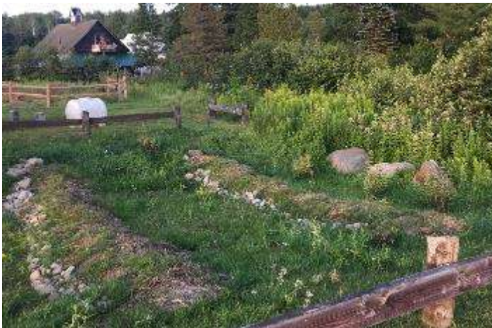
Figure 29. Picture of the restoration of an unused boat ramp and one of 4 rain gardens installed at Seymore Lake by the NorthWoods Stewardship Center Work crew in 2019.
