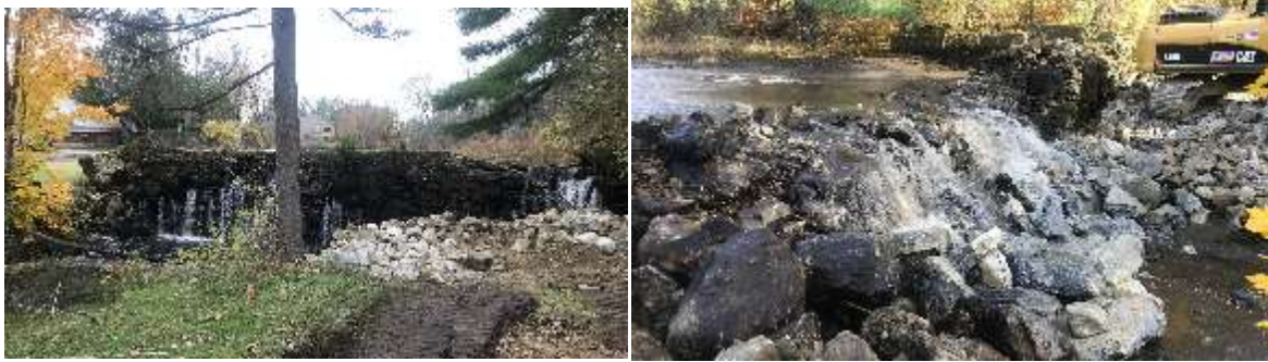
Figures 11. Partial breach of the Dunklee Pond Dam in Rutland City on 10/30/2019. Left: Before breach, Right: during breach.
