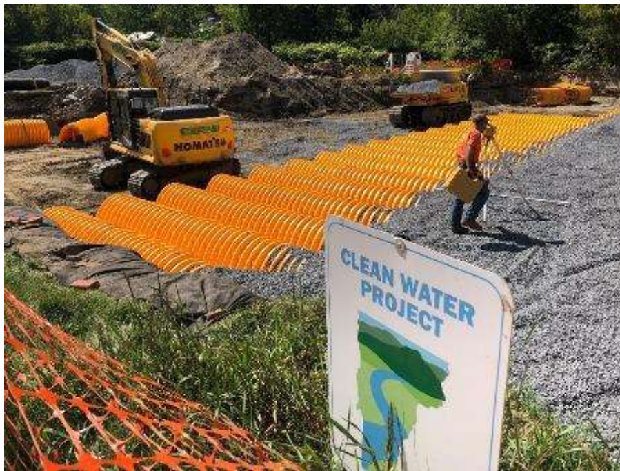
Figure 19. Stormwater from Water St in Northfield diverted from Dog River into Stormwater treatment chambers
