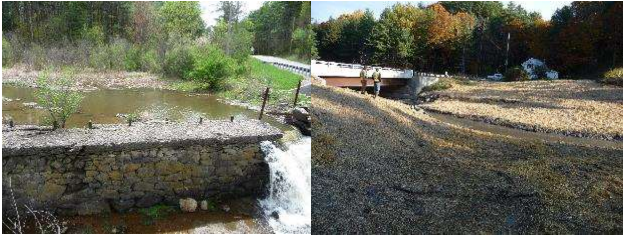
Figure 12. Mill Pond Dam before and after dam removal and restoration project
