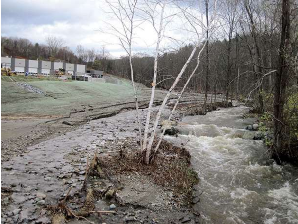
Figure 14. Beecher Hill Brook floodplain restoration project post construction (photo credit: Jessica Louisos).
