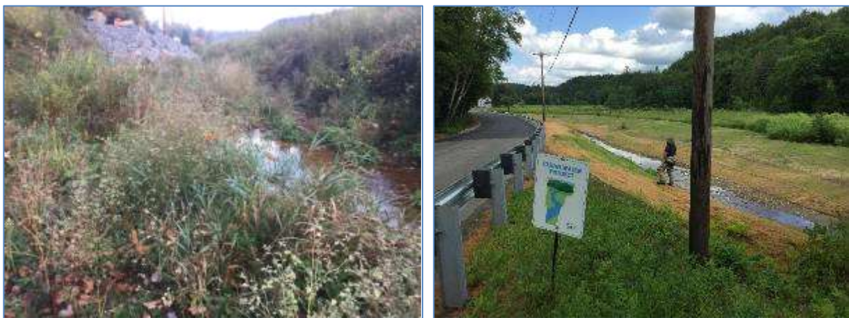
Figure 18. Deeply incised flood chute with riprap on roadside bank (left). Restored flood chute stabilized and vegetated (right). Vegetation on riprap will decrease pollution from road stormwater runoff and eventually provide shade and habitat for aquatic organisms.
